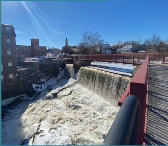
Spicket River Dam in Methuen
