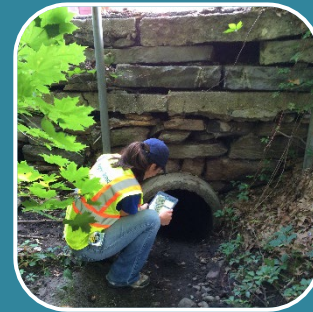
Stormwater Infrastructure Maintenance
