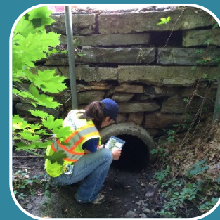
Stormwater Infrastructure Maintenance
