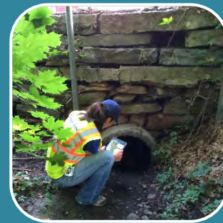
Stormwater Infrastructure Maintenance
