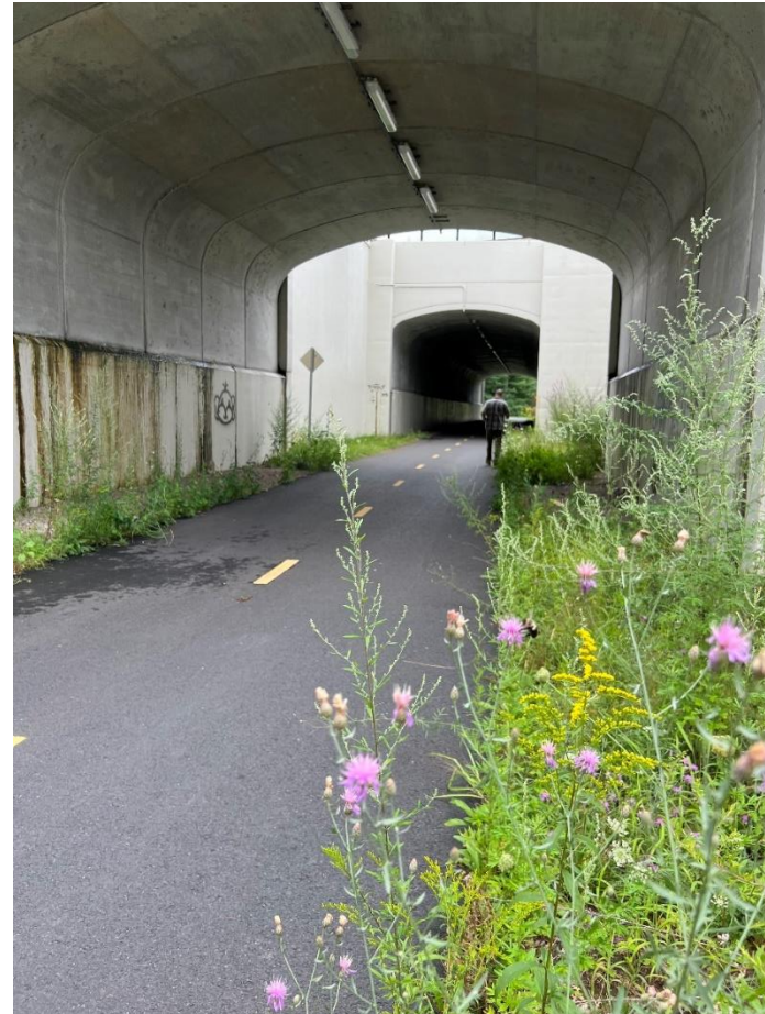
Shared use path tunnel under I-95.
