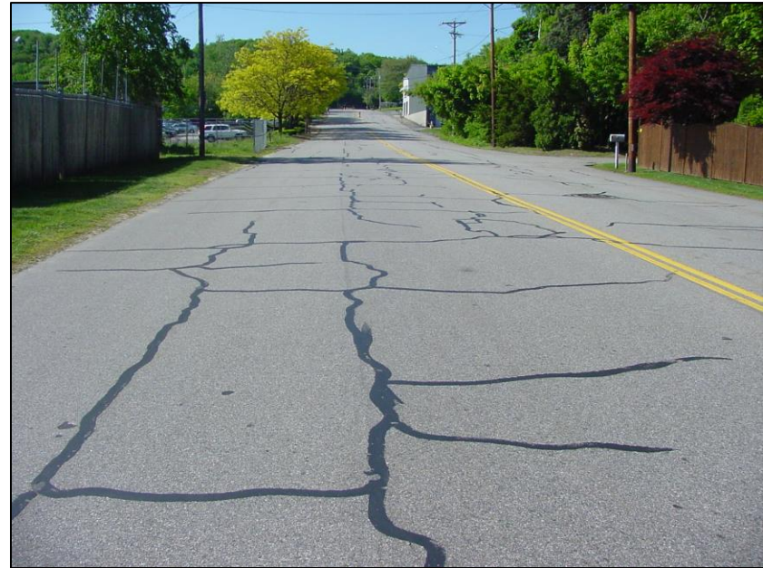
Photo: Example of crack seal applied on a road.
