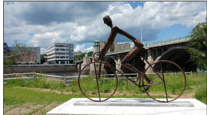
Photo: Replacement of the Basiliere Bridge (shown in background) is programmed in the 2024 element of the TIP.
