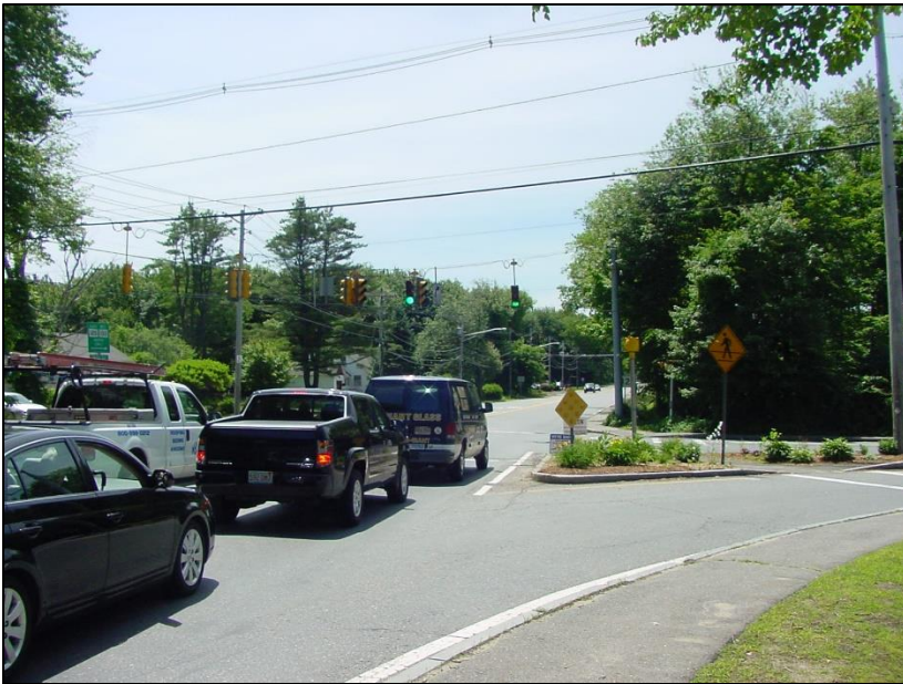
Photo: Route 125 at Massachusetts Avenue in North Andover is the site of a federally funded project.
