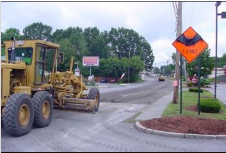
Photo: Reclamation of a roadway.
