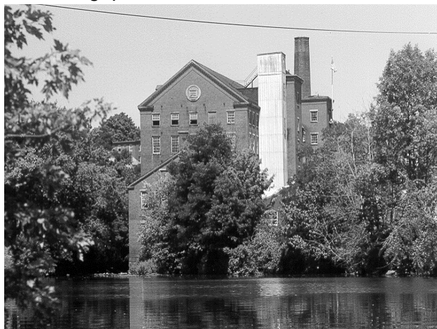
Lower Millyard in Amesbury. Source: MVPC
