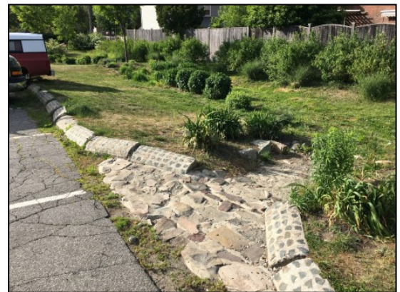
Example of green stormwater infrastructure
