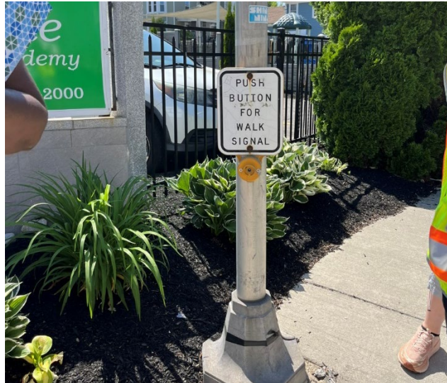
Figure 38. Broken Pedestrian Push Button at the Intersection of Jackson and Haverhill.
