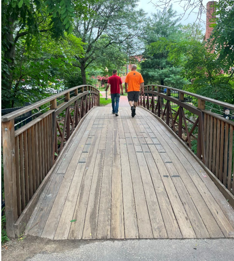
Figure 44. Pedestrian Bridge over the Powwow River in Amesbury, MA.
