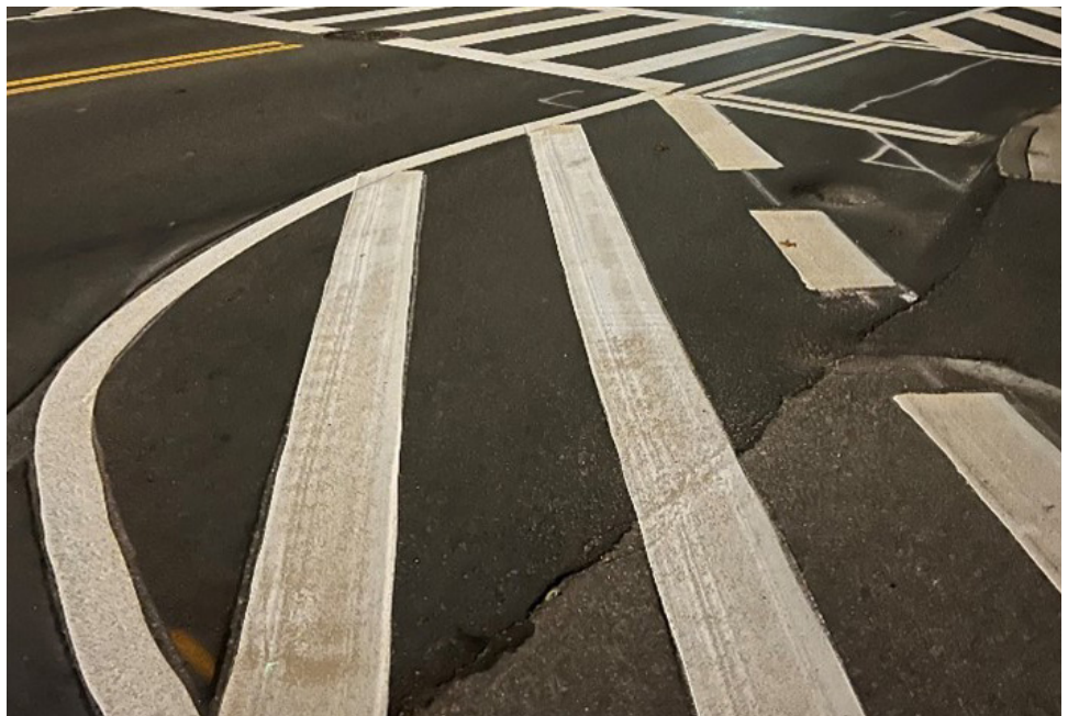
Completed Thermoplastic Markings in Groveland
