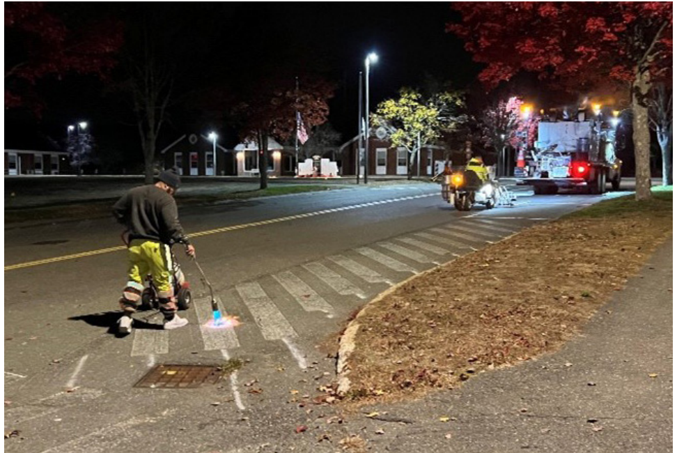
Preparing Recessed Areas for Thermoplastic in Groveland
