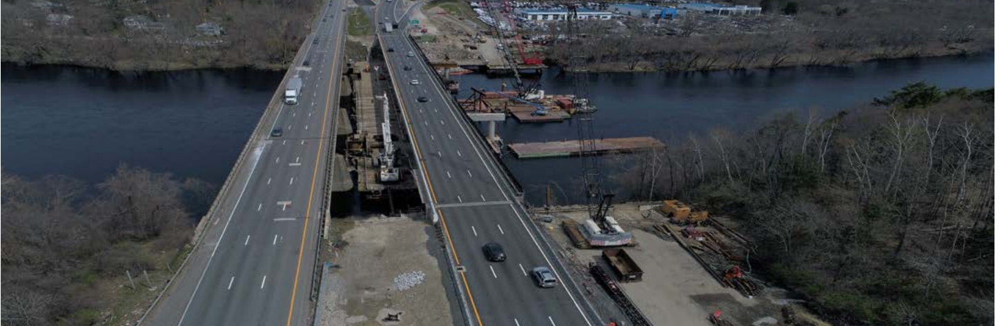
Route 495 bridge replacement, Photo by MassDOT April 2020
