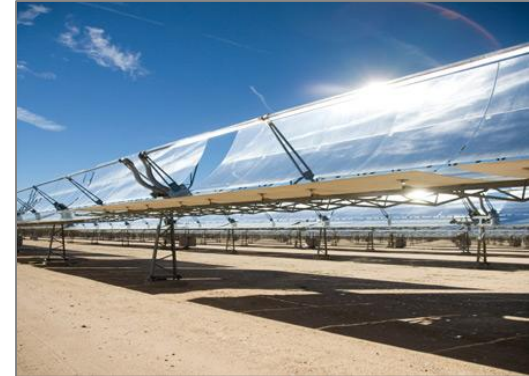
Concentrated Solar Power
