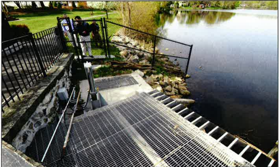
Water enters the new drainage system through the crest gate at the southeast corner of Ell Pond
