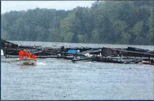
Destroyed Boat Slips – MacKenzie's Landing Marina, Amesbury
