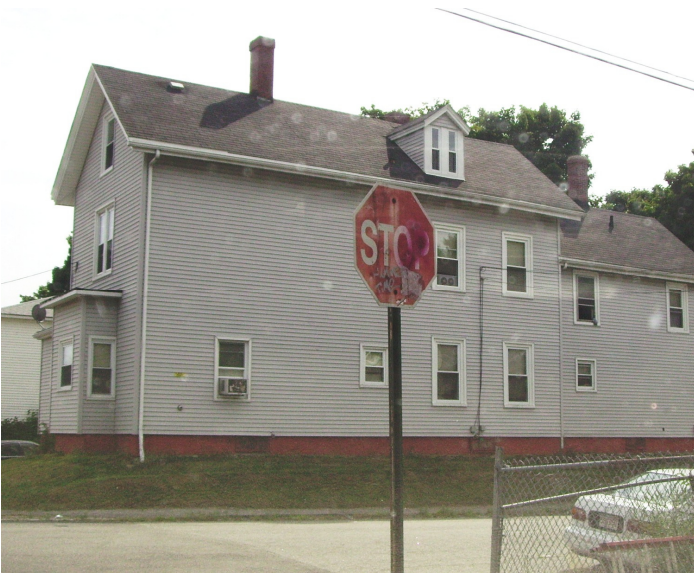
Lower Acre streets are marked by many damaged or missing signs.
