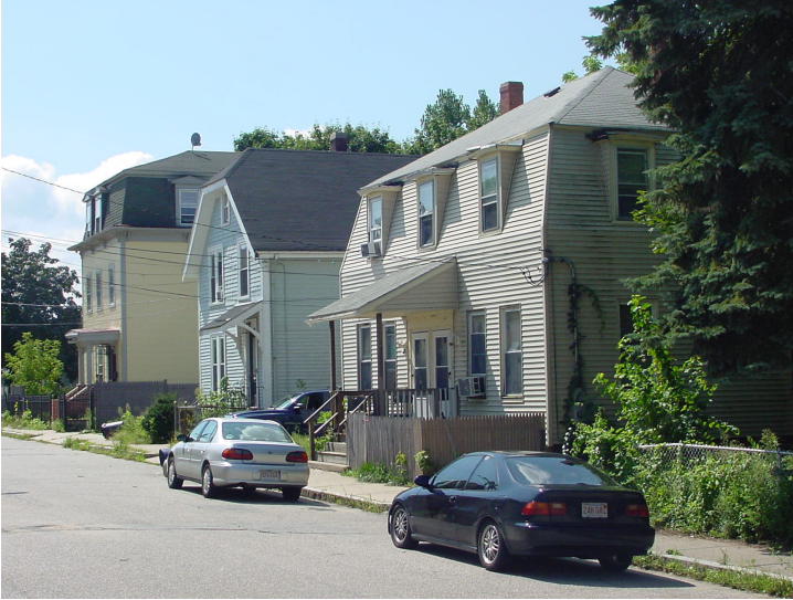
Homes in the Lower Acre are in a variety of states of repair. Many code violations and unsafe conditions were found in a survey of exterior conditions.
