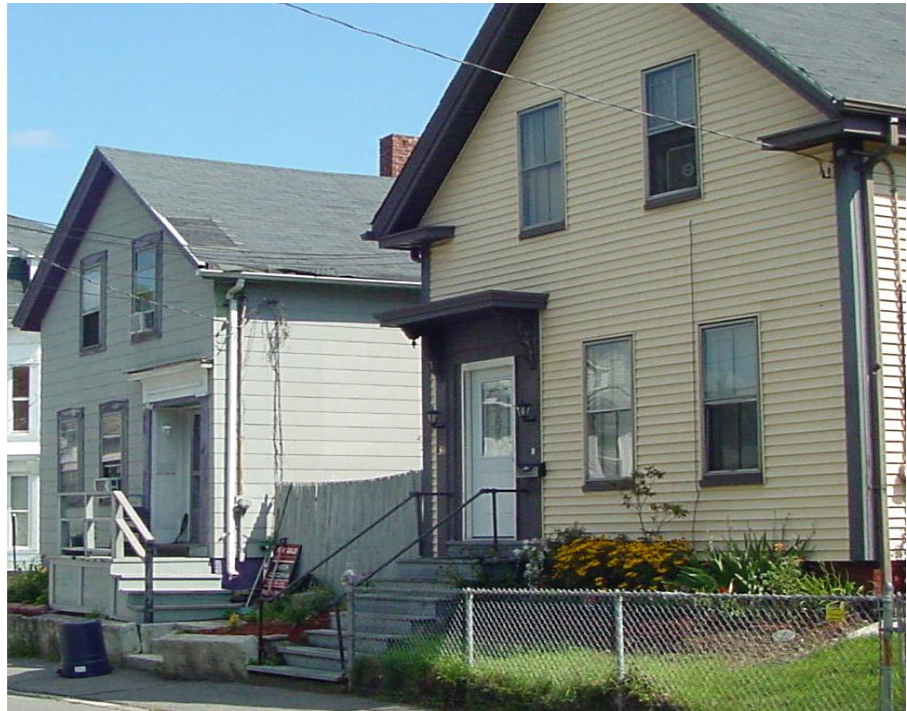
In the Lower Acre, well-kept homes and poorly-maintained structures often stand side-by-side.
