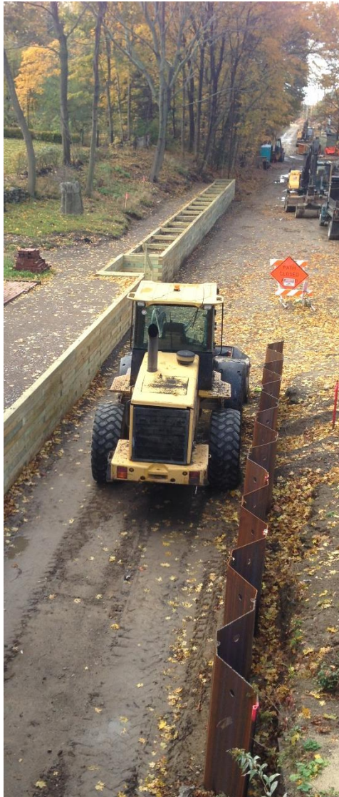
Image: Construction of the Clipper City Rail Trail in Newburyport.
