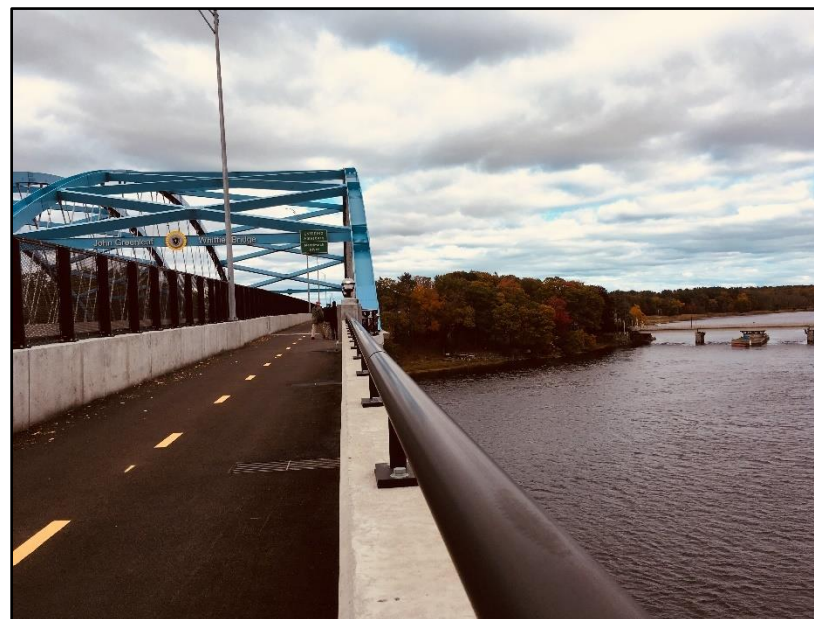
Photo: The Garrison Trail along I-95's Whittier Bridge opened in October 2018.
