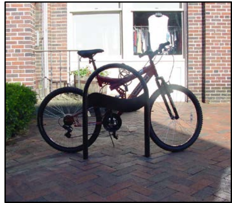
Photo: Racks should support bikes in two places.
