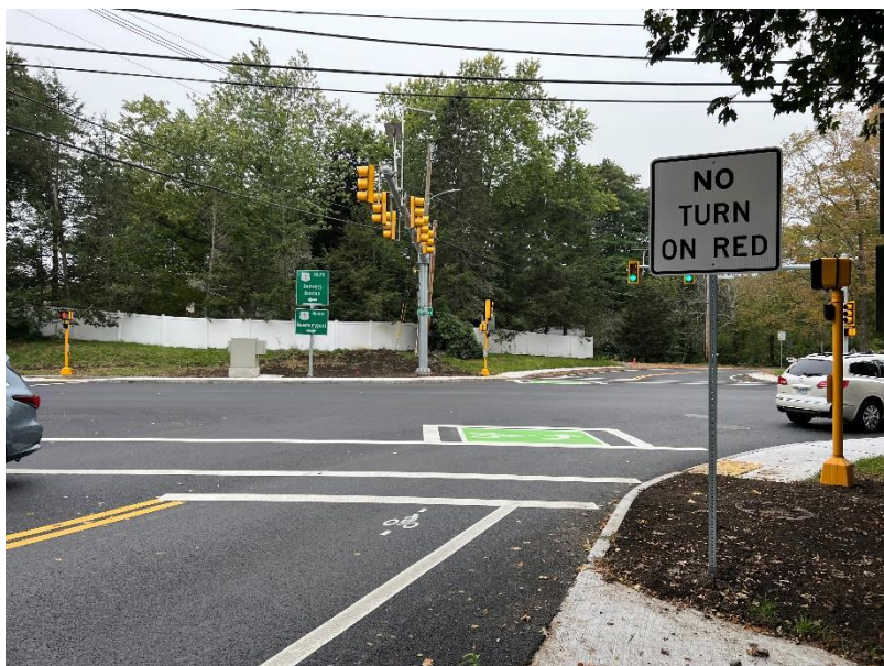
Route 1 and Glen Road, Rowley
