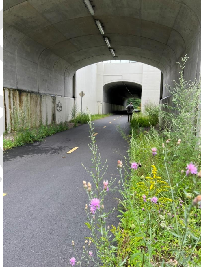
Shared use path tunnel under I-95.
