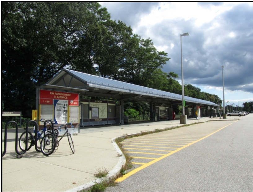
Rowley Commuter Rail Station
