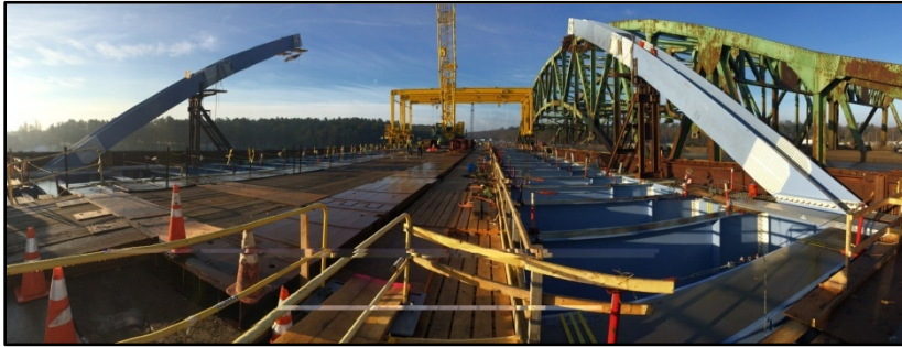
Photo: Whittier Bridge, MassDOT
