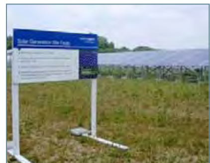
National Grid, Haverhill
