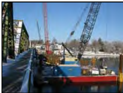
Bates Bridge Reconstruction - photo by Ken Cadman, HNTB
