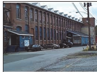
Stevens Street Mill, Haverhill
