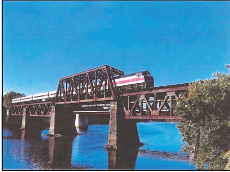
MBTA Merrimack River Bridge, view west
