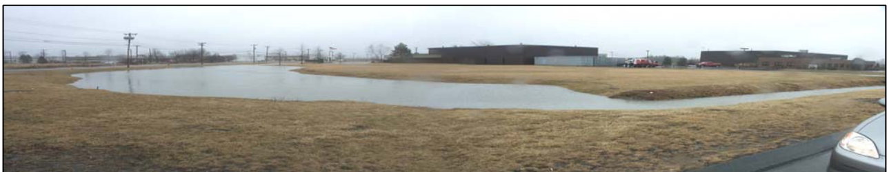
Zampell Detention Basin on the corner of Malcolm Hoyt and Stanley Tucker Drives April 2, 2004
