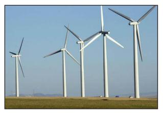
stand-alone turbines, either built separately, or grouped together to form a wind farm. These turbines can be connected to a grid to provide utility-scale electricity to a region, off-setting the use of fossil fuels normally used to generate electricity. Wind turbines consist of a tall tower with a fan-like rotor that turns with the force of the wind, which turns a shaft inside the turbine that spins a generator to make electricity.
