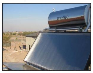
created by warming up these solar collectors to heat water in the tank. The hot water rises to the top of the tank and pumped down into the house or building where it's attached. While solar thermal hot water collectors are a cheap and efficient way to harness the heat energy from the sun for a practical use in the home, almost all systems require a backup hot water heater on cloudy days or days without direct sunlight such as winter months.
